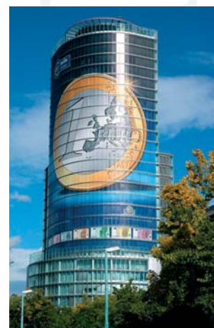
The NBS building clothed in a mega billboard.
